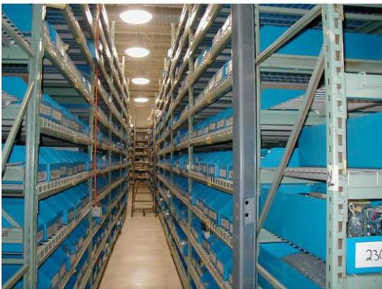
Three sizes of Milform® bins were decided on with two different lengths to fit 36" and 48" wide shelves. Two bin widths were decided on (23.50" and 11.75") to accommodate the variety of parts sizes, yet maximize shelf length. The depth decided on was 8" in all bin sizes in order to increase the number of shelves per rack.
